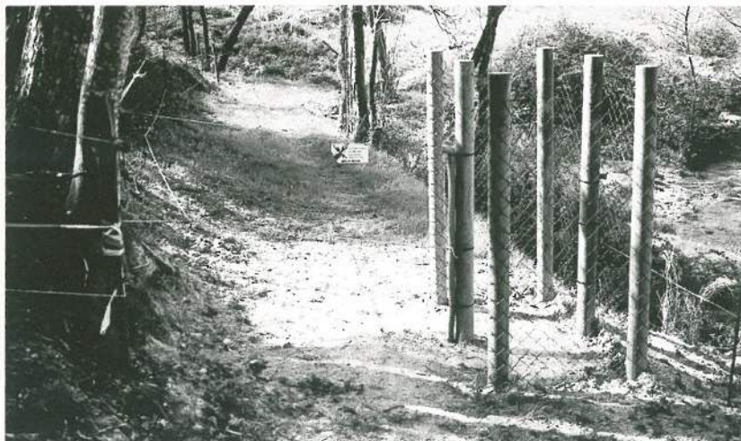
Installation de chicanes.
